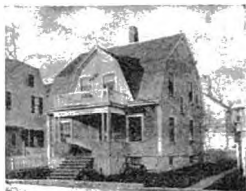
A No. 22 IDEAL Boiler and 240 ft. of 38-in. AMERICAN Radiators, costing the owner $115, were used to Hot-Water heat this cottage.
