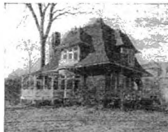
A No. C-242 IDEAL Boiler and 555 ft. of 38-in. AMERICAN Radiators, costing the owner $250, were used to Hot-Water heat this cottage.
